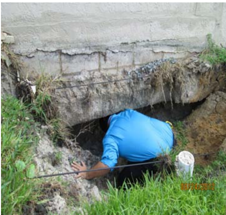
Checking under the foundation of a house
